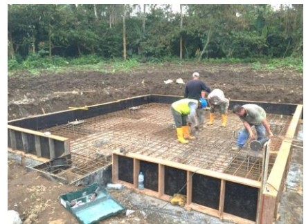
FORMWORK AND MESH OF ELEVATED WATER TANK
