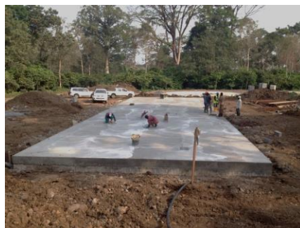
SLAB FOR PURIFICATION PLANT
