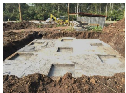
SLAB FOR ELEVATED WATER TANK
