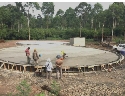
SLAB FOR DRINKING WATER TANKS
