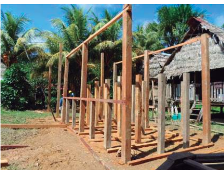
CONSTRUCTION OF STILT HOUSES
